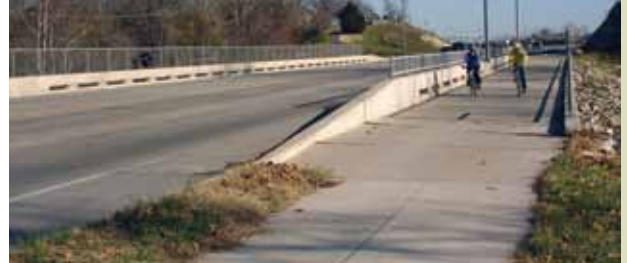
East Broadway Bridge before and after highway improvements were carried out according to the street design standards
